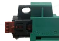
The disconnect is now in the "off" position. It should be locked out using between 4.5 and 6 mm padlock.
